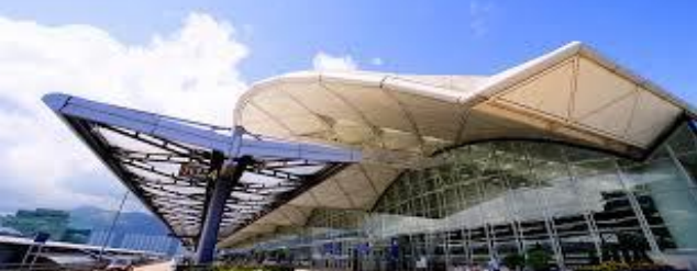
Hong Kong Inter. Airport
